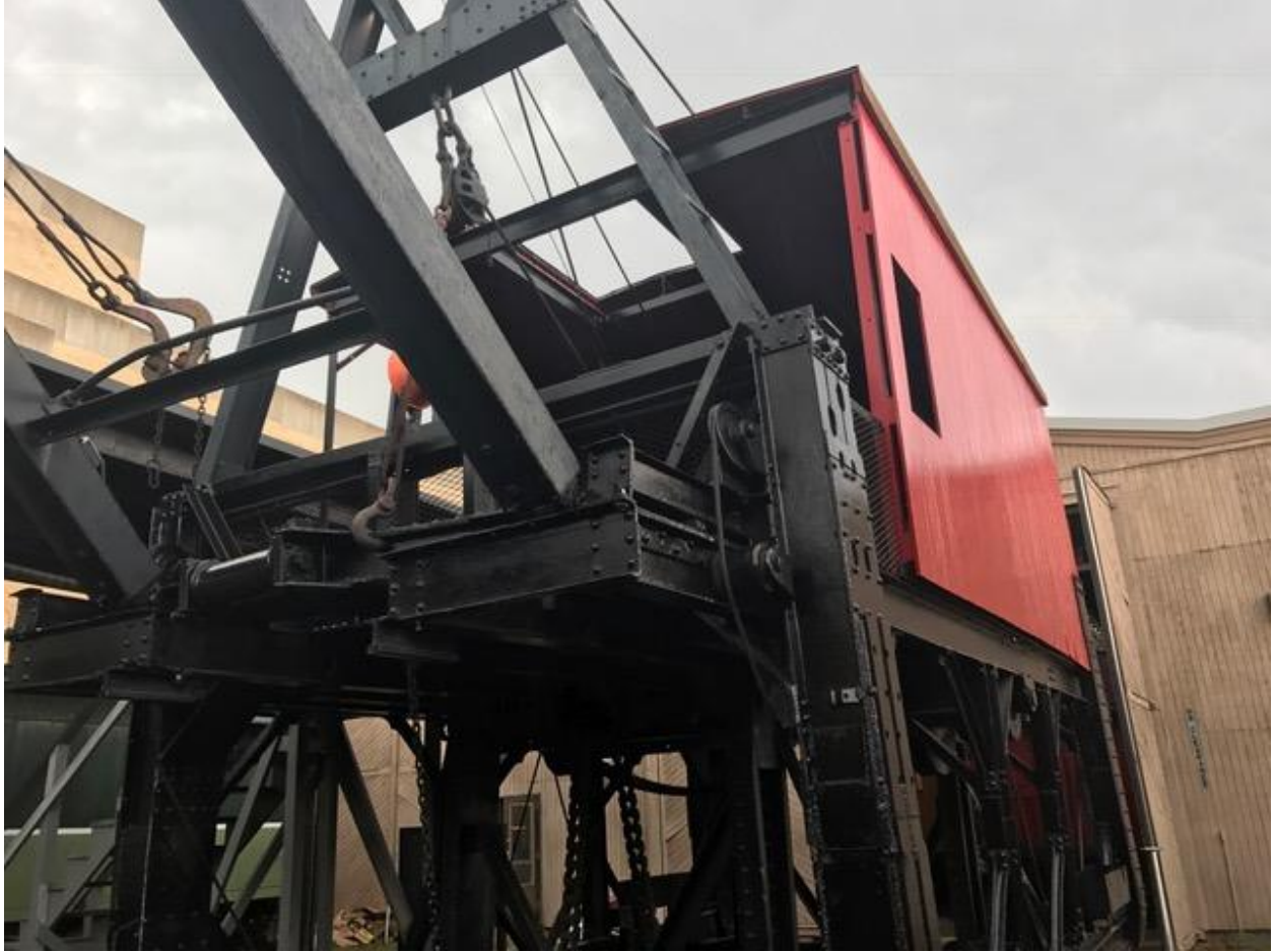
Log loader house in the raised position so empties could pass underneath.
