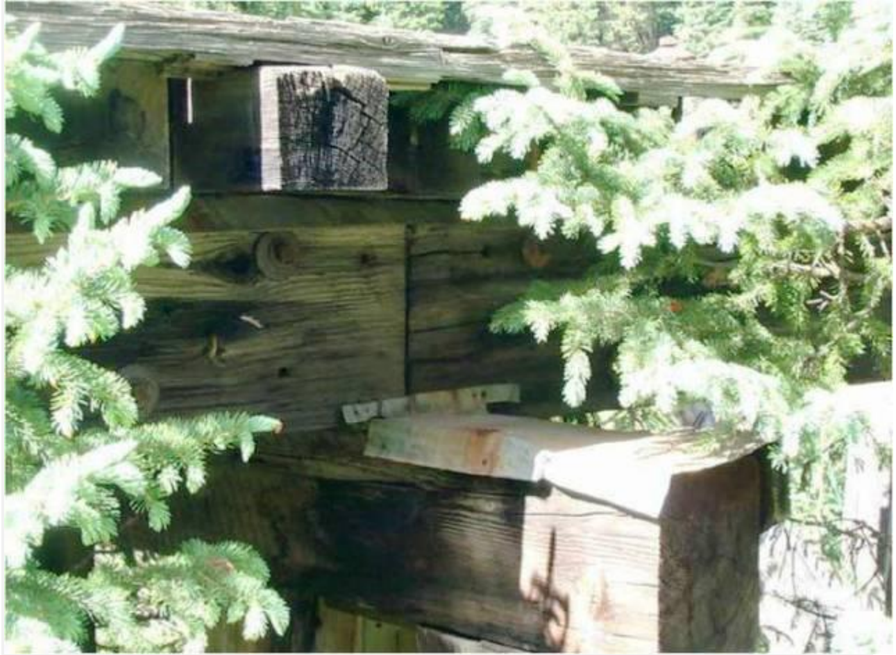
Photo 5 - Stringer / Bent Detail
