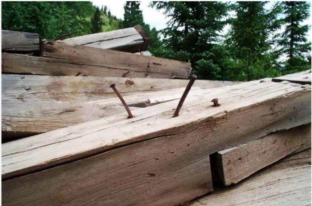
Photo 8 - Spliced Sills and Boat Spikes (Bridge 44A)
