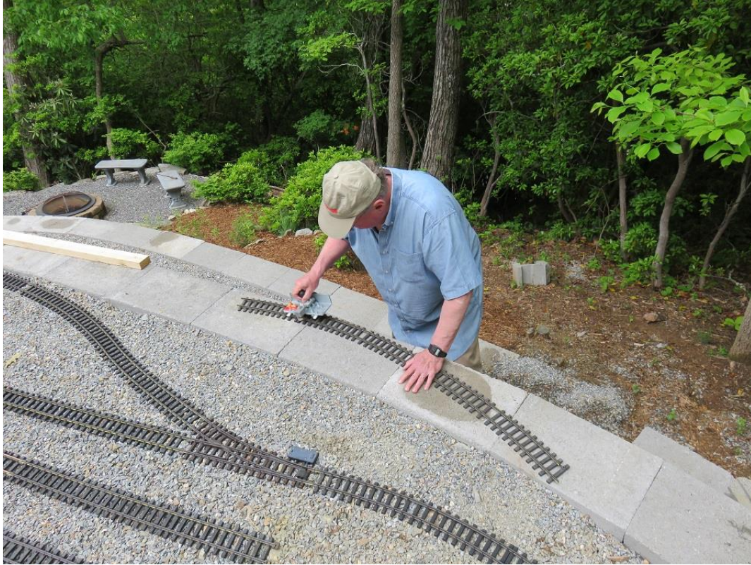
Larry Williams and Doc Watson manned the railbenders while Todd Jacobus and yours truly worked the Dremel tool and installed the rail clamps to join the track sections.
