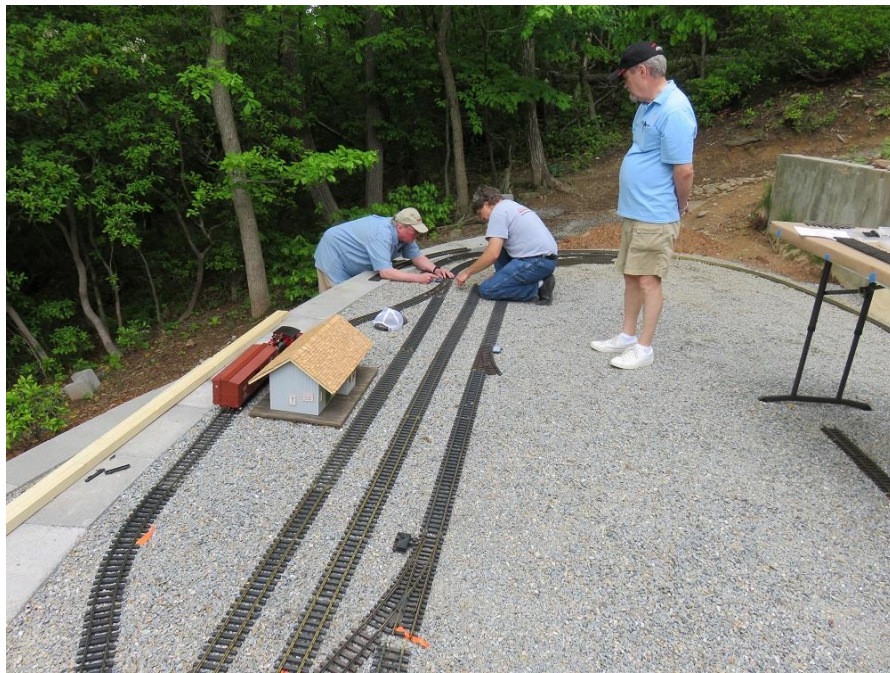
Doc Watson takes a short break after installing the passing track and mainline around the station to supervise Larry and Todd's progress connecting the outer radius curves.
