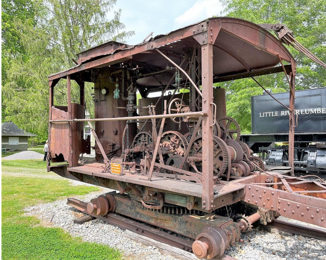
American Hoist and Derrick Log loader
